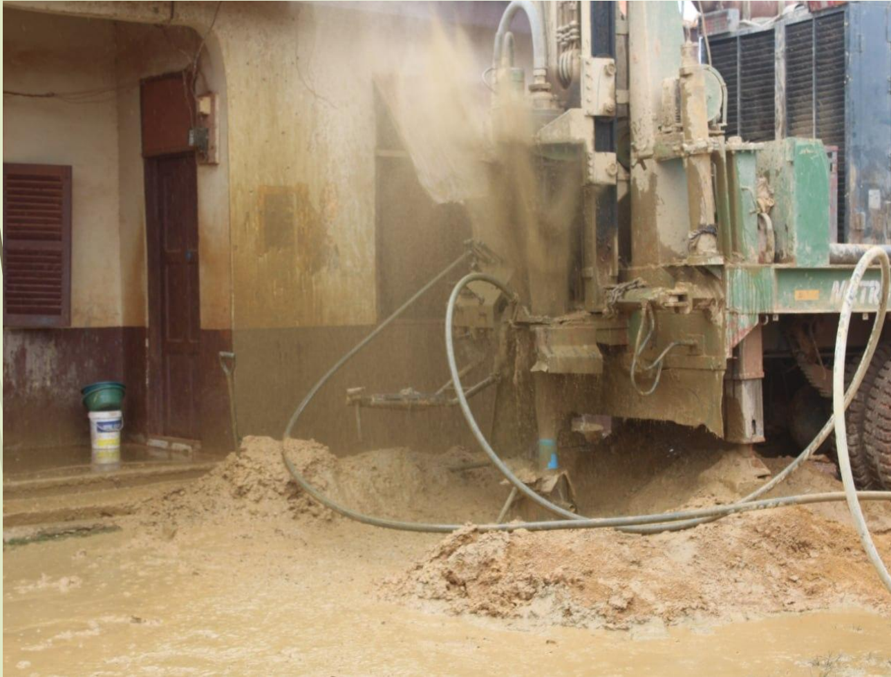
Drilling of deep borehole
