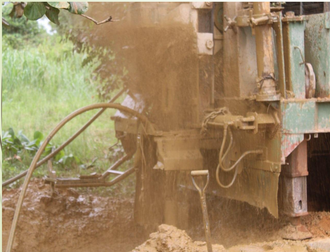
Drilling of deep borehole
