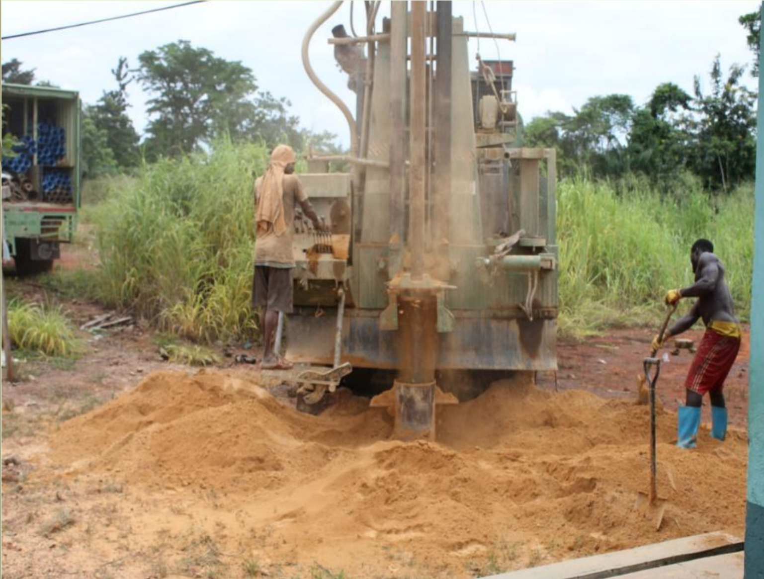
Drilling of deep borehole
