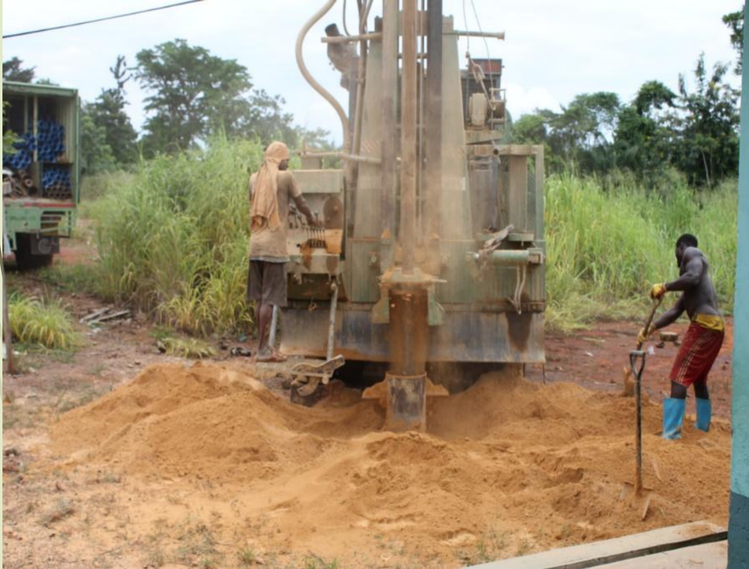
Drilling of deep borehole
