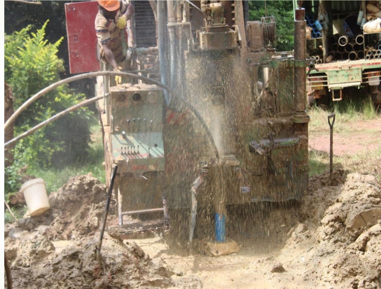
Drilling of deep borehole
