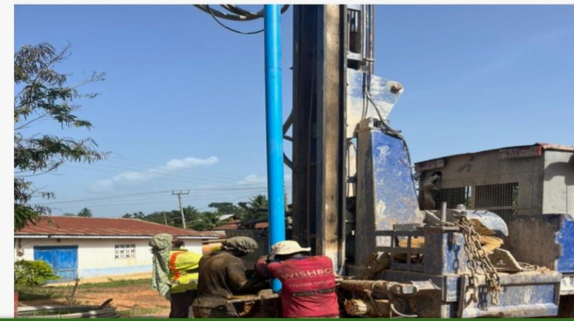
DRILLING OF DEEP BOREHOLE AT ADDAIKROM KWAOSO D/A BASIC
