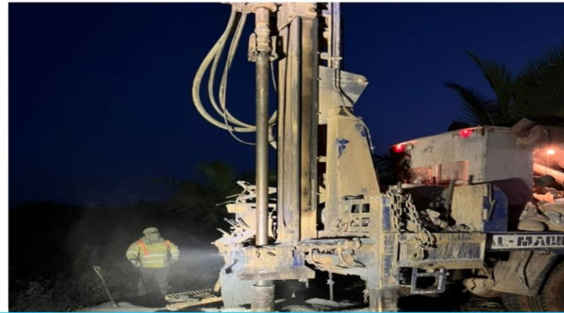
DRILLING OF DEEP BOREHOLE AT DEBRA TAABOSERE CHIP COMPOUND
