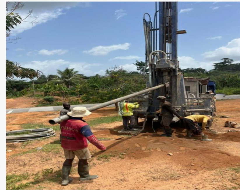
DRILLING OF DEEP BOREHOLE AT ADDAIKROM KWAOSO D/A BASIC
