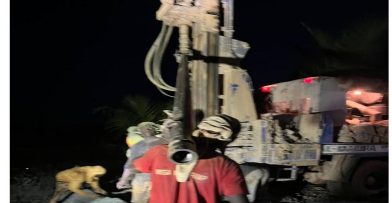
DRILLING OF DEEP BOREHOLE AT FENASO KWAADOKROM D/A BASIC
